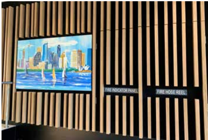
Installation method. Battens are back screwed through MDF panel.
