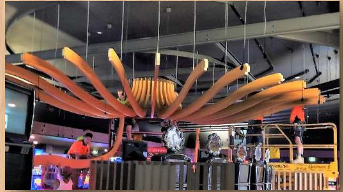
Installation of curved Ecolite beams—Brisbane Lions @ Springwood
