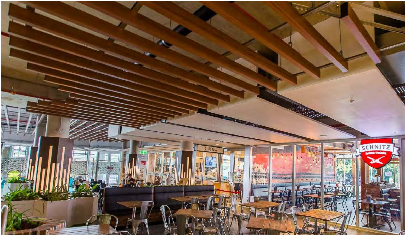
Newmarket Village Food court area. Digitally printed aluminium beams in Heritage Walnut.
