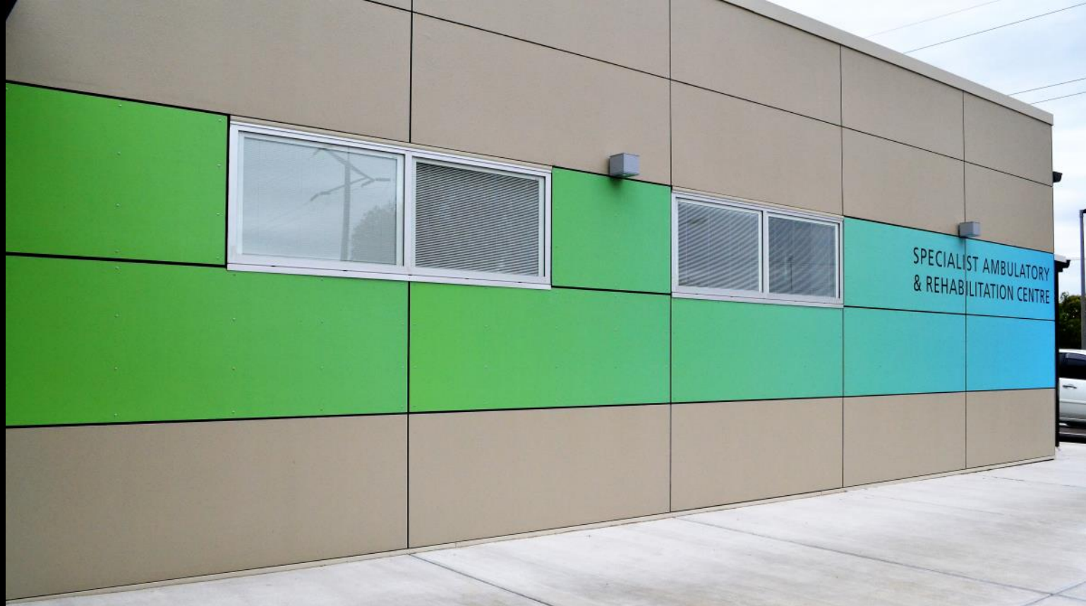
Modbury Hospital—Adelaide Architect GHD Builder: Built Environs Product: CFC panels digitally printed and anti-graffiti coated.
